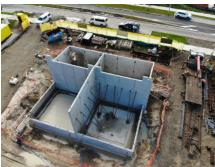
To keep the substation watertight, the outside of the basement was sealed with a quality waterproofing system and drainage was installed around the perimeter to divert the ground water to a nearby creek.
