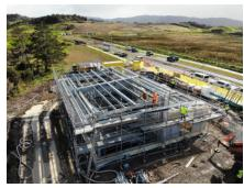
The building features a control room, switch room, fibre room and two large-scale transformer bays, which required installation of custom-designed 5.8m-tall precast wall panels and full-height aluminium ventilation louvres.
